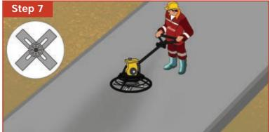
As soon the concrete has hardened sufficiently not to be damaged power float the surface with steel blades until smooth and slightly shiny.
