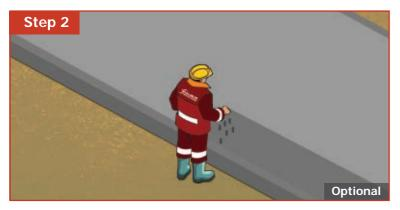
After bleed water has evaporated, immediately reinforce edges by spreading hardener by hand along a 150 to 200mm edge and finish using wooden trowel.
